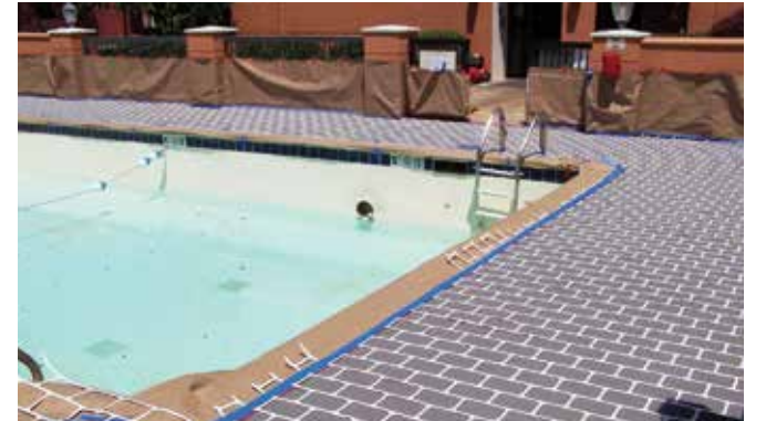
Stencil pattern is rolled out before applying accent color.
