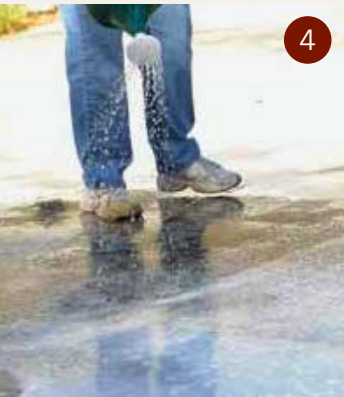
Acid etching can open concrete pores.
