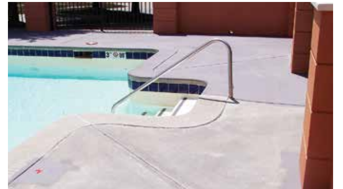
Base coat application begins.
