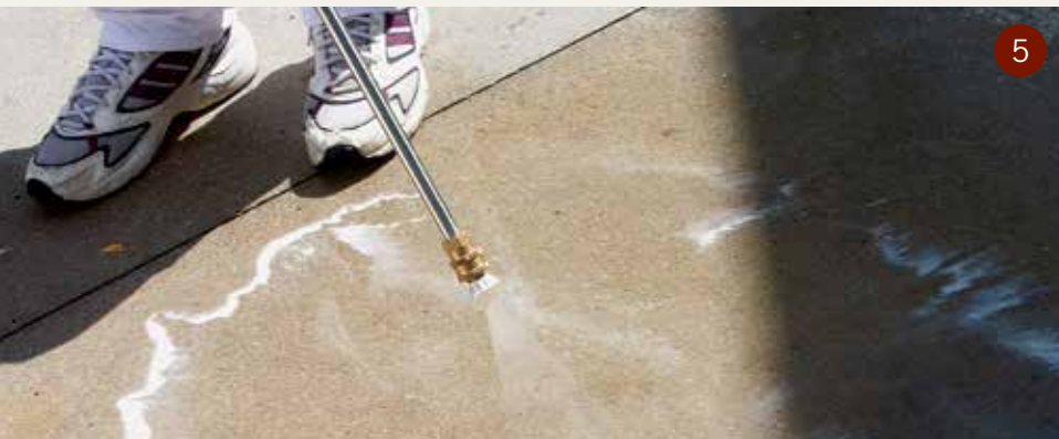
Proper preparation ensures bonding of your protection system to the substrate.
